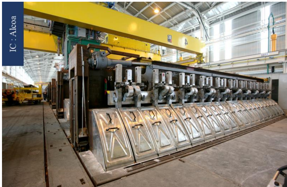
Figure 2-2 : A prepared reduction cell ready for energisation
