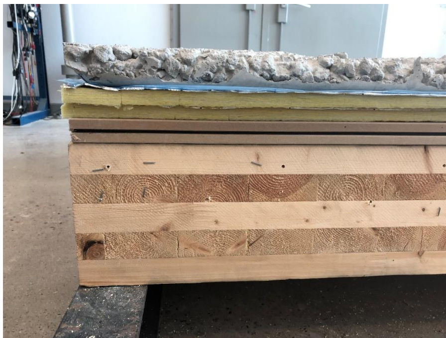
Figure 5.2: Compositions of the floating floor. Materials from the top to the bottom: concrete; insulation layers; gypsum boards; CLT panel.
