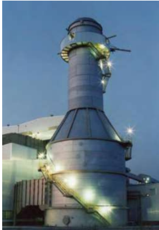
Figure 2.5. Sodium based absorber at the Alcoa Massena East smelter [3]
