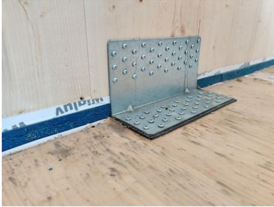
(a) Resilient interlayers between bearing elements and under bracket.
