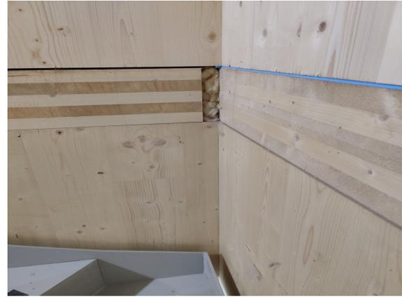
(b) CLT-junctions in a staircase with resilient interlayers.
