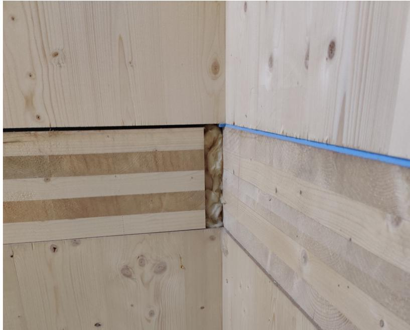
Figure 5.1: Junction with cross-laminated timber and elastomers as viscoelastic interlayers.
