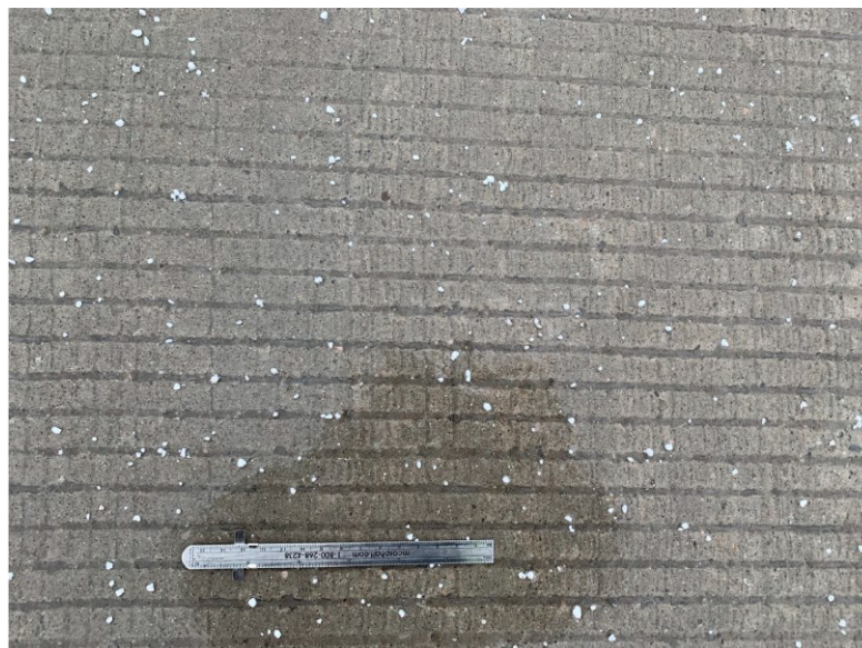
Figure 4-2: Sodium formate (NaFo) over a concrete pavement runway surface, illustrating the application concentration used at Mirabel airport, Québec.
