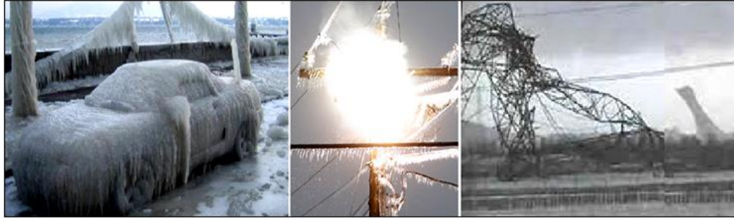
Fig.1.1. Atmospheric icing ( left ), flash over in iced overhead transmission lines ( center ) and destroyed transmission pylon ( right ) caused by accumulated ice, the Quebec ice storm 1998 [3-5].
