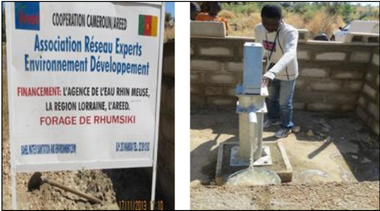
Figure 2. Construction effective du forage
