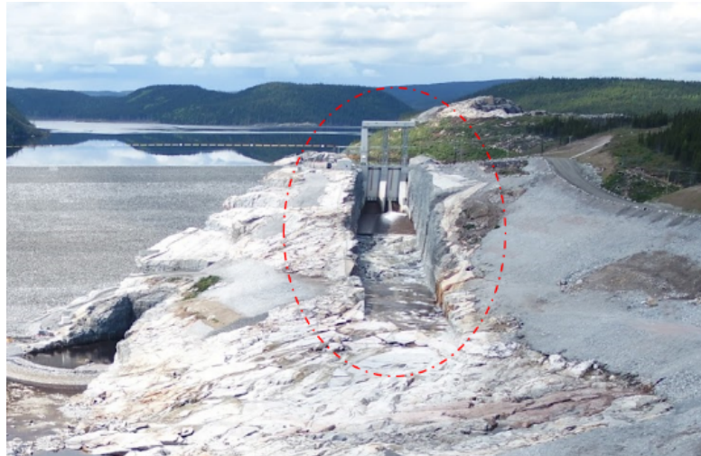
Figure 4.1 : Photograph of Romaine-4 spillway outlined in red (© Hydro-Québec)
