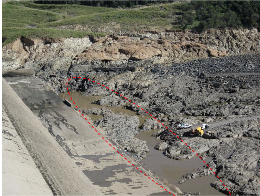
Figure 2.4 : Condition of the Paradise Dam spillway following the 2013 flood. Dashed red lines outline the eroded area. Modified from Lesleighter et al. (2016)
