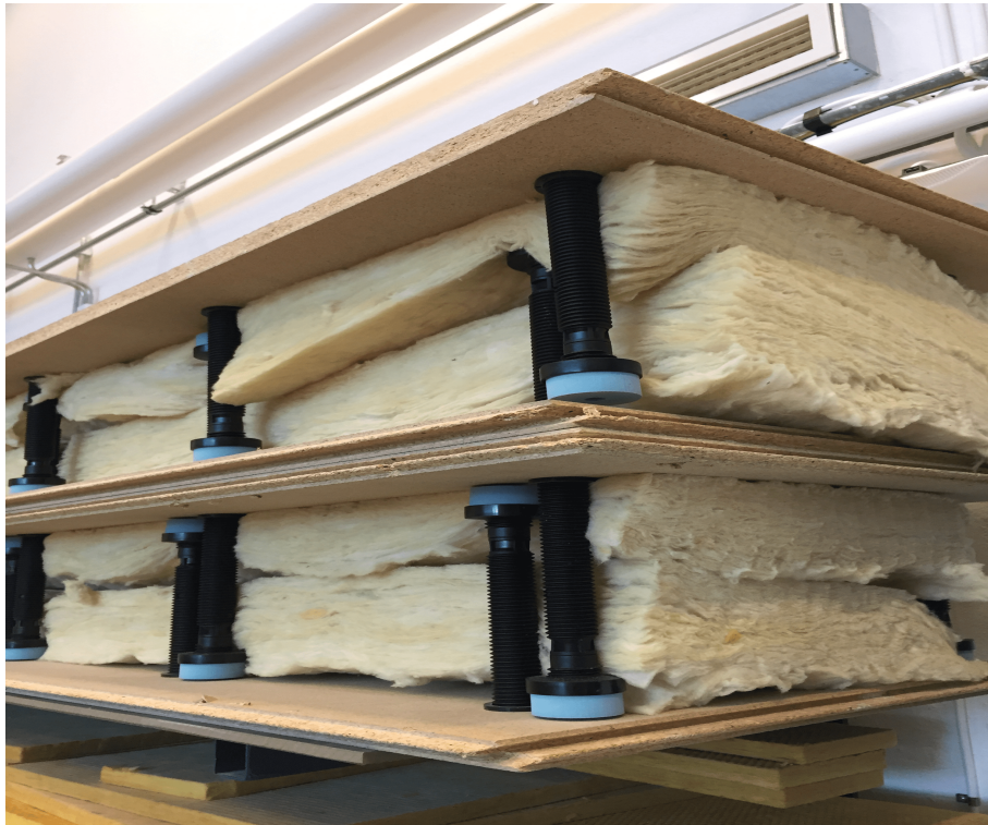
Figure 4.5: A dry-rise solution system that uses boards on top of point supports with integrated resilient interlayers.
