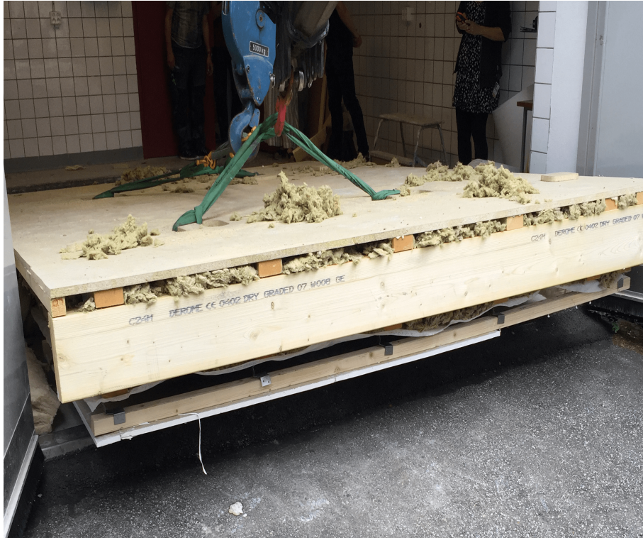
Figure 4.4: A wooden floor structure is installed in the laboratory of Lund University to quantify the sound insulation measurement.
